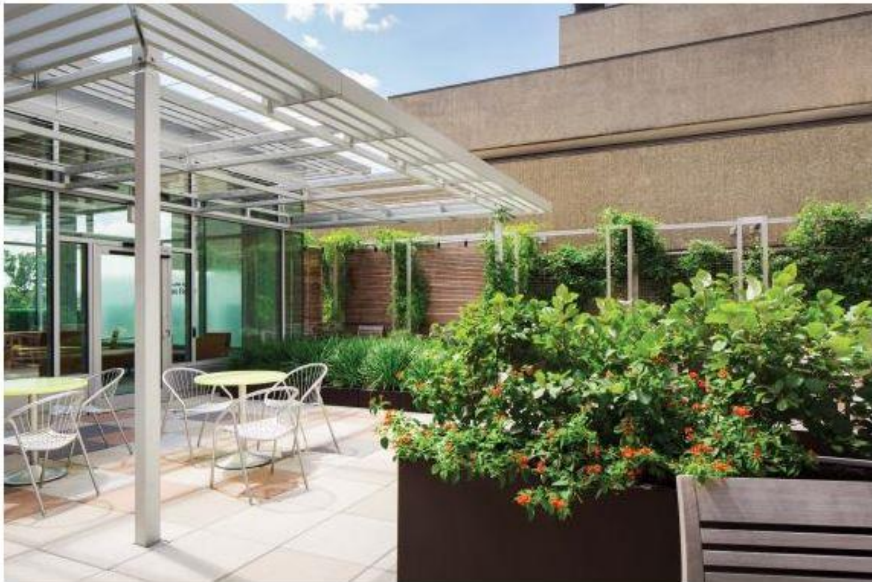
Danbury Hospital, Danbury, Conn. Bronze Award. Custom wood and metal trellis structures with strategically placed plants create shading and privacy around seating areas. Photo: Mark Weinberg.
